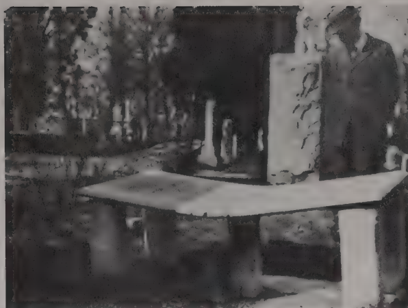
Figure 9.37 Marble bench that sagged with time under the influence of gravity.
