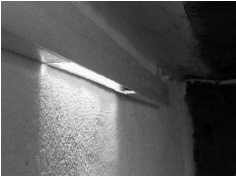
Figure 4-16. Light exit, cut into wire channel
