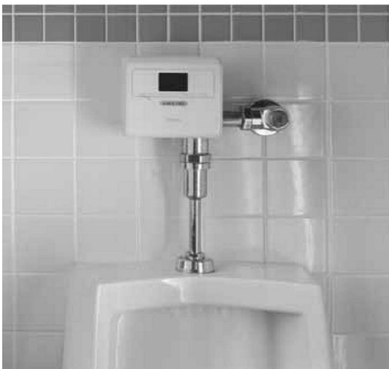
Fig. 1: Installation of the automatic flush system
